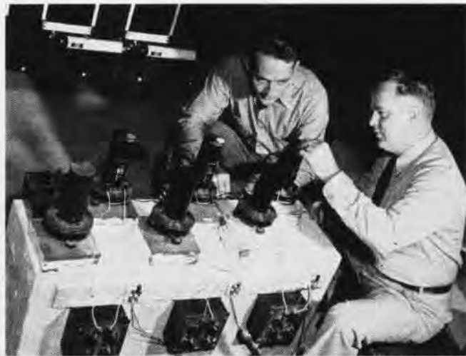
ADJUSTMENT IS BEING MADE TO GALVANOMETER IN RECORDING VAULT
