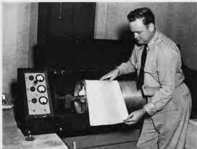
A 'TRACE' RECORDS NORMAL EARTH TREMORS ON PHOTOGRAPHIC PAPER
