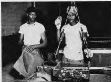
DEGREASING PARTS BEFORE DIP IN COMPOUND
