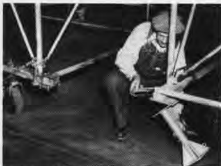
HINGE MAKES IT POSSIBLE TO LOCK LEGS UP
