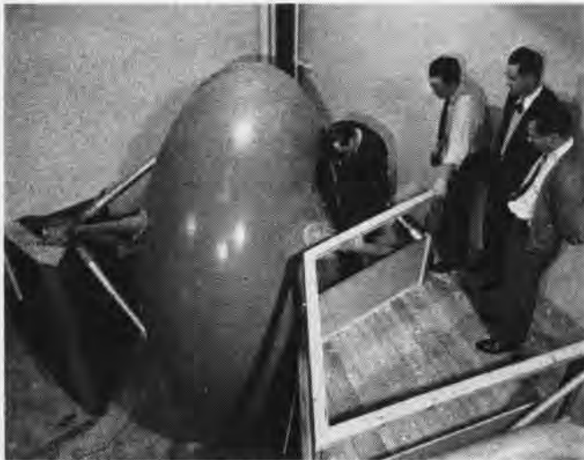
MOCKUP OF GONDOLA WHICH WILL SPIN SUBJECTS AROUND CENTRIFUGE
