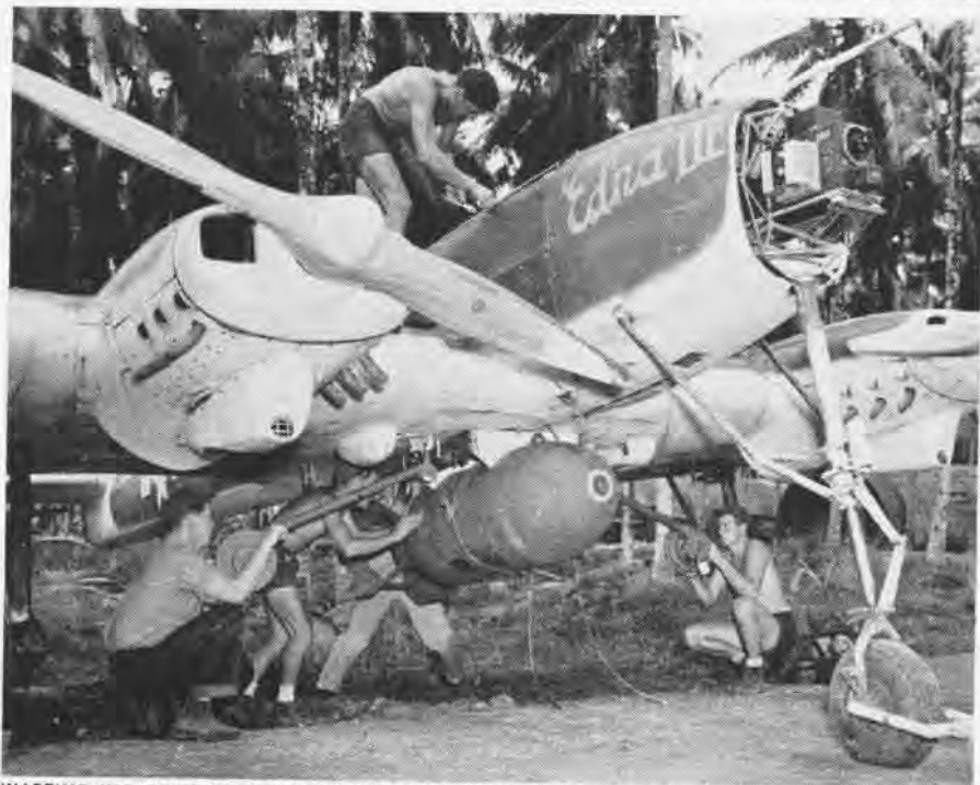
WARTIME USE OF TDR-1 REMOTE-CONTROL PLANE WAS TO DROP 2,000-POUND GP BOMB ON JAPS
