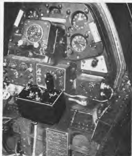
DRONE CONTROL UNIT IN F7F'S REAR COCKPIT
