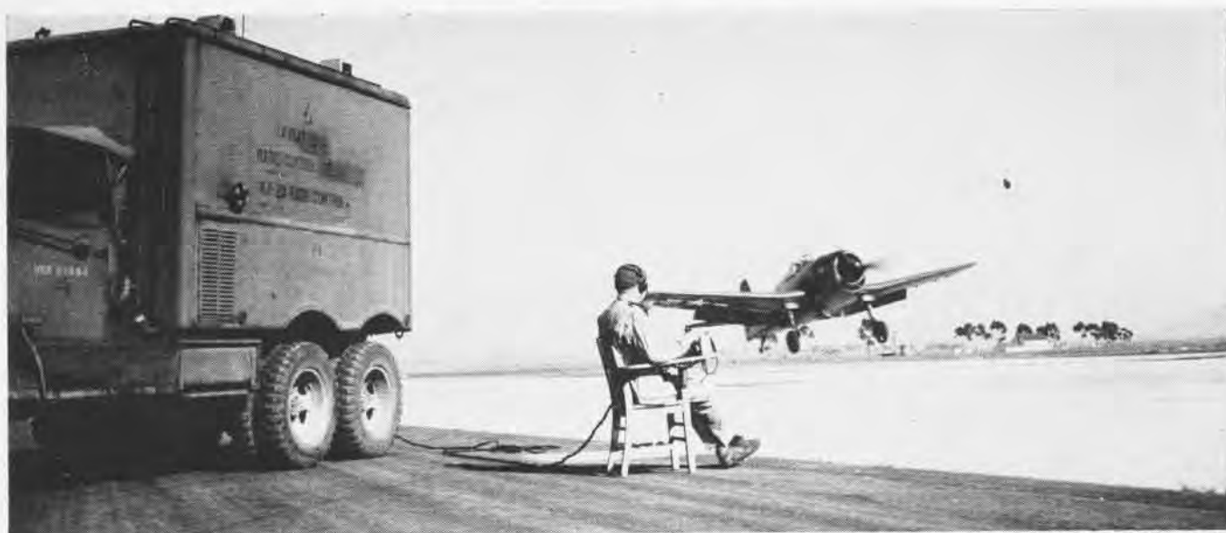
GROUND CONTROL OFFICER ON OPERATION CROSSROADS BRINGS IN RADIO-CONTROLLED HELLCAT DRONE; PLANES FLEW THROUGH ATOMIC CLOUD
