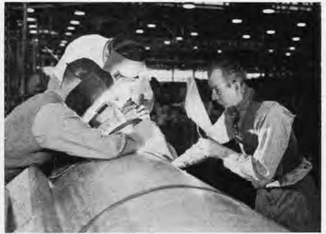
2 WELDING ONE of the rocket's fuel tanks at Martin plant is closely supervised; oxygen and alcohol power Viking
