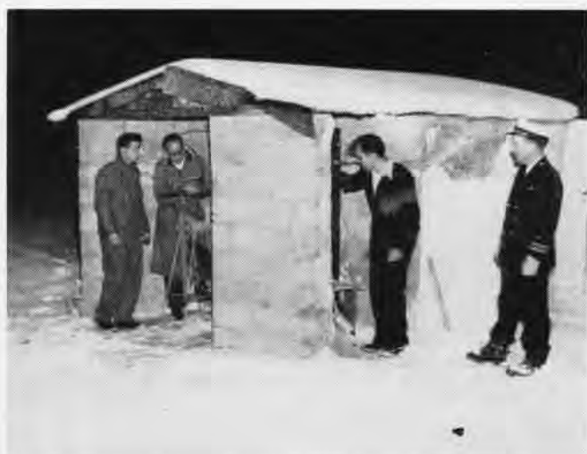
ICE AND snow can't stop VAU-9-15's Benepe, Goddard, Struble and Baske in preparing for rocket motor tests in their cement block unit
