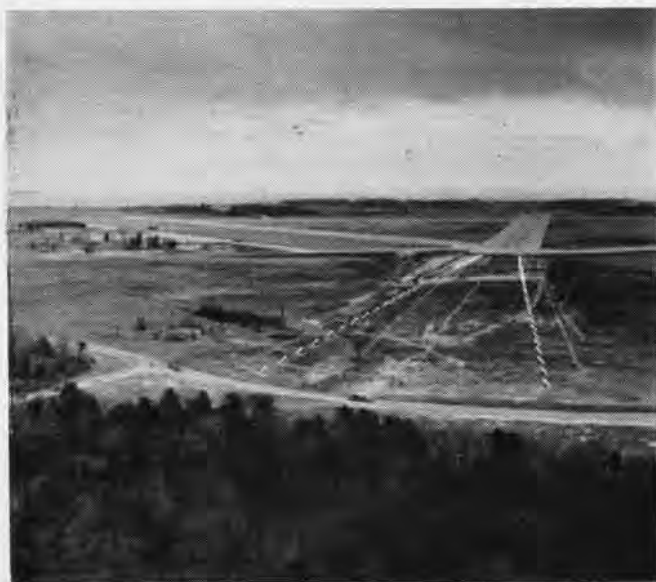
MANY OF THE tests on the airport slope line approach light system were performed at Arcata, Calif.; here is the Paruxent installation
