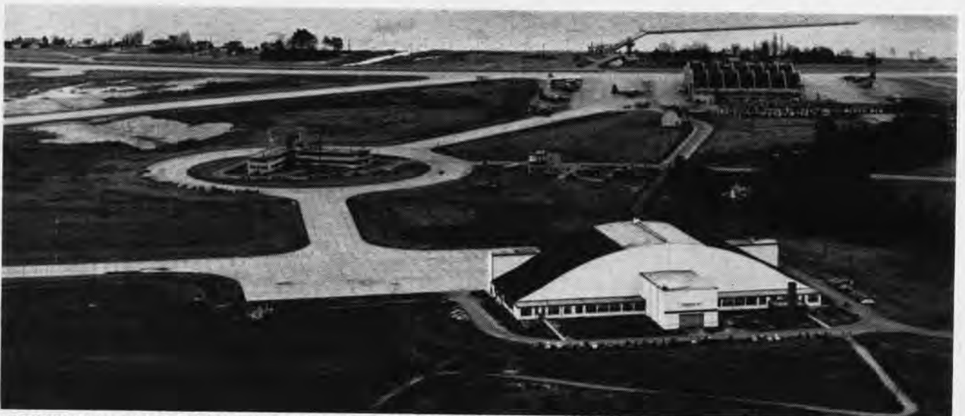
ELECTRONICS TEST AREA AT NATC PATUXENT RIVER, MD., IS SHOWN HERE: HANGAR IN FOREGROUND IS SHIELDED, COVERS AREA OF FOOTBALL FIELD
