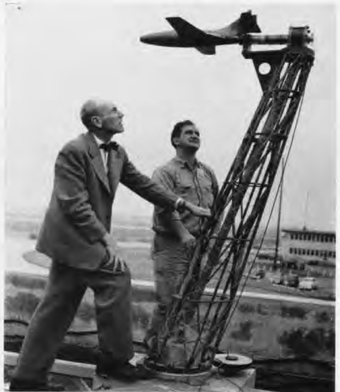
MONEY IS SAVED by antenna section by using models; Section Head R. L. Hensell, and J. E. Canetti at model mounted for radiation test
