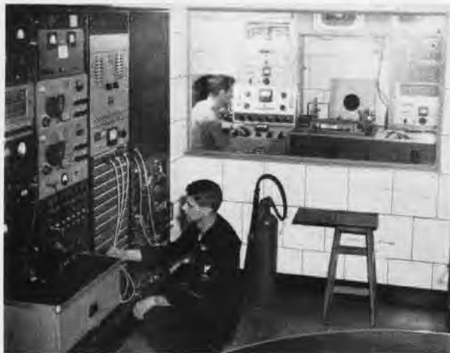
RECORDING EQUIPMENT in tower at Electronics Test is operated by J. R. Carr, AL3, at panel, and E. Leonard, AL1, sitting at console
