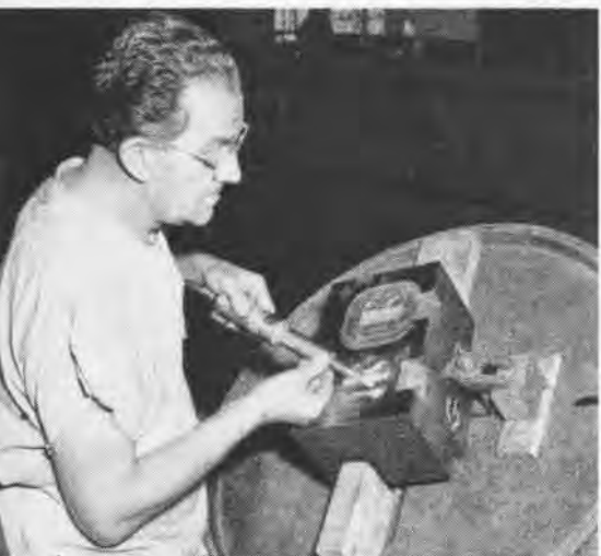
MACHINE SHOP —NAF's Yaeger finishes impression in die blocks for barrier cable clamps
