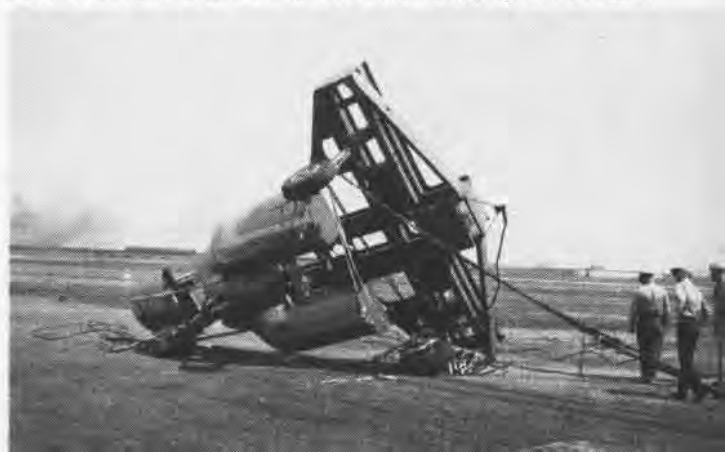
TESTING EXPERIMENTAL barriers at NAMC—Dead load configured like aircraft is swung over on side after engaging barrier cables
