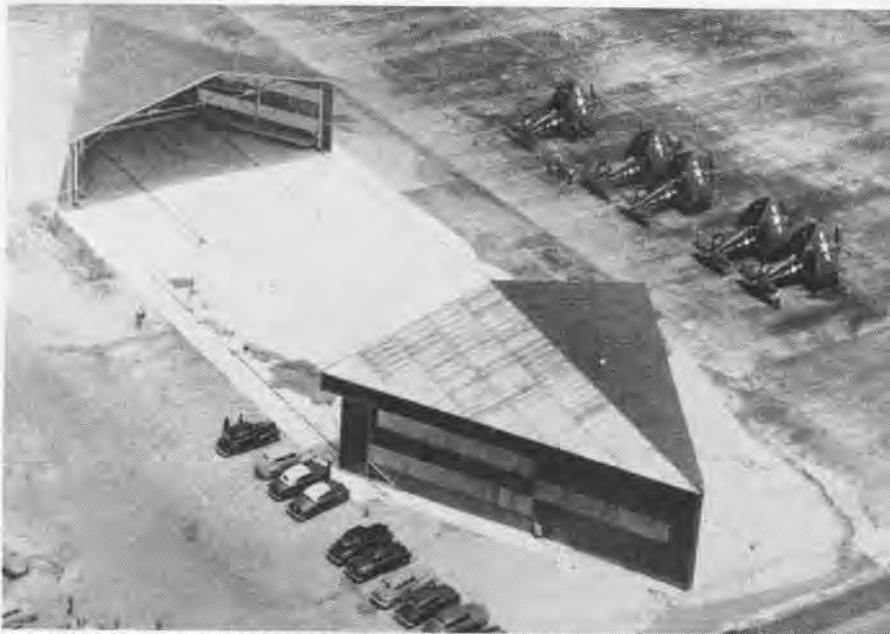
MOBILHANGAR AT CHERRY POINT IS SHOWN HERE FULLY EXTENDED, READY TO RECEIVE AIRCRAFT
