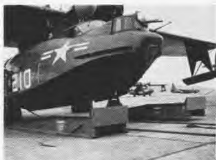
ONE RAMP IN POSITION, SECOND BEING MOVED
