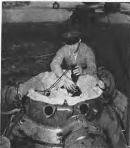
FASRON 112 man redrills oil passage before installing reworked couplings in the engine.
