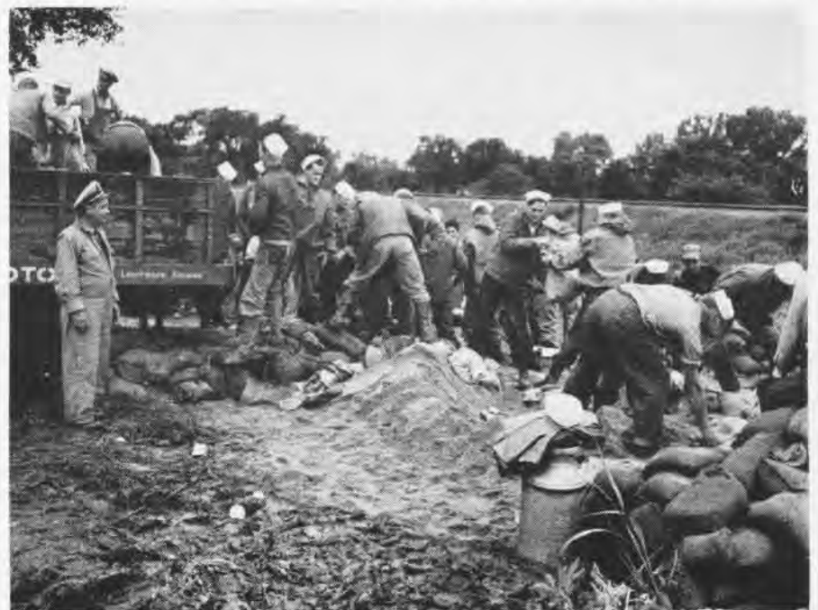
LCDR. FREEMAN WATCHES SAILORS FROM NAS OLATHE WORK HARD TO PROTECT LAWRENCE LEVEE
