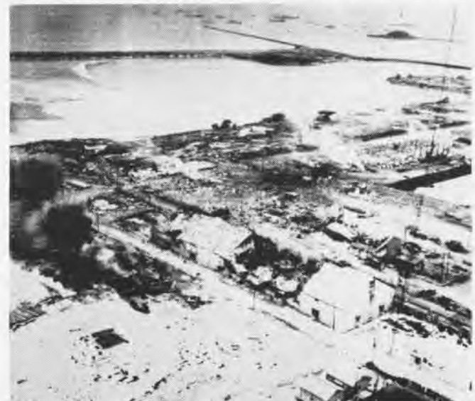
BATTERED KOREAN port facilities in this radiophoto indicate possibilities of reconnaissance radio facsimile transmissions
