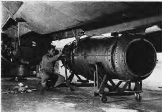
J-48 MOUNTED UNDER B-29 IS READIED FOR MOUNTING OF AFTERBURNER
