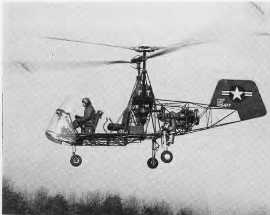
STRIPPED-DOWN KAMAN HELICOPTER WITH GAS-TURBINE POWER: NOTE SMALL POWERPLANT SIZE
