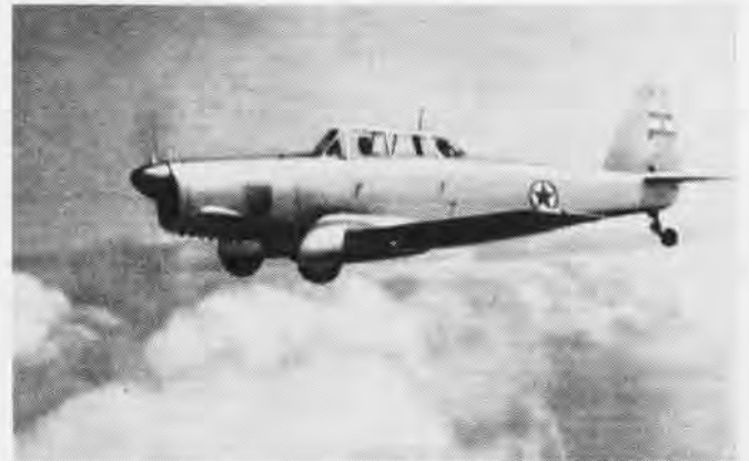
YUGOSLAV 213 TRAINING PLANE HAS PARTIALLY RETRACTING WHEELS
