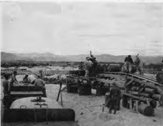
RODGERS' gravity fuel system in operation; ramp permitted filling fuel trucks far faster than by hand pumping plan once used
