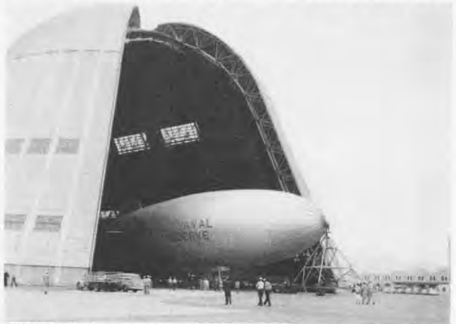
THE GOOD old days came back to NAS Moffett Field with this G-ship. Hangar 1 was built originally as homeport for the Akron and Macon, handled 12 blimps this size
