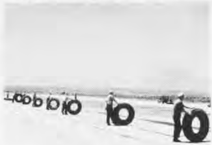
JURY-RIG FIELD ARRESTING WIRE USES TIRES
