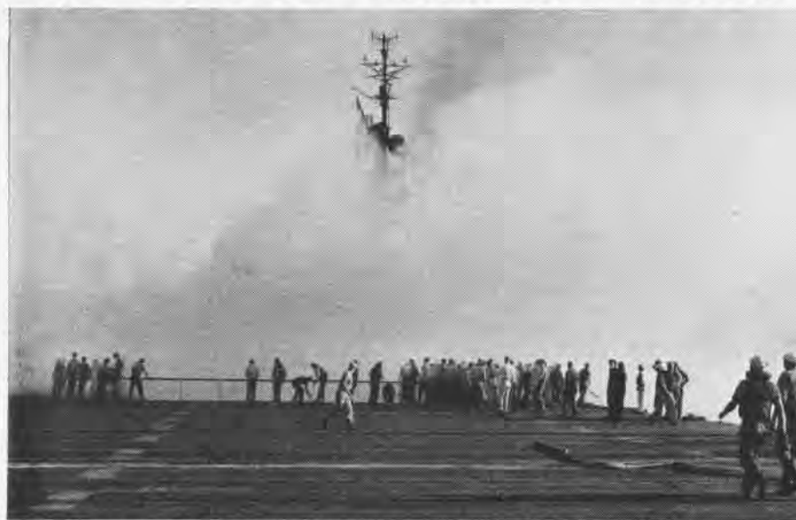
THICK SMOKE POURS OUT OF #3 ELEVATOR AS CREWS ON HANGAR DECK FIGHT FIRE ON THE BOXER
