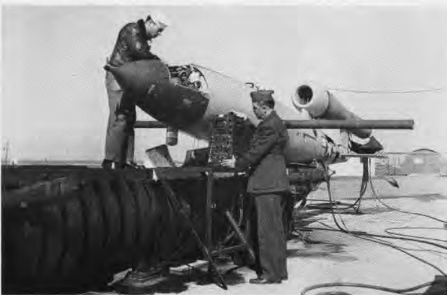
NAMTC PT. MUGU'S FACILITIES TEST VARIOUS GUIDED MISSILES LIKE THIS PULSE-JET FOR NAVY
