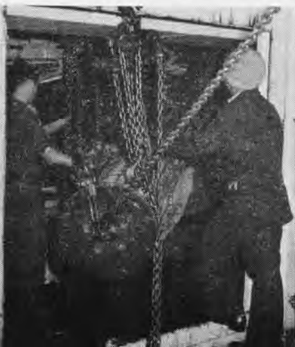
10-FOOT HOLE IN BULKHEAD REQUIRED FOR JOB
