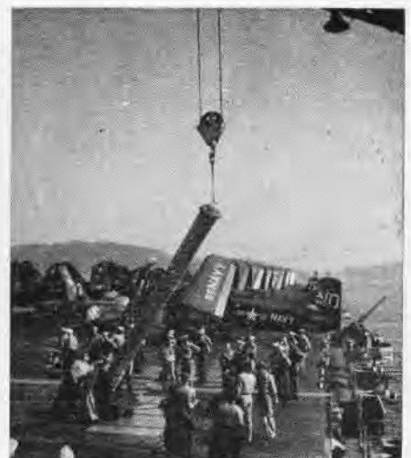
CYLINDER STARTS DOWN BOMB ELEVATOR SHAFT
