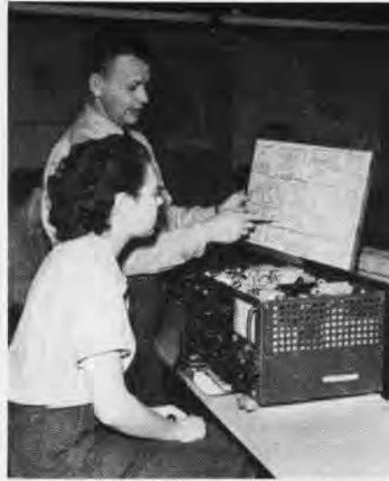
PEHOSH, ATC, helps WAVE Newby search for calibration on frequency indicator circuit
