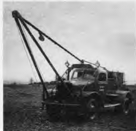
DUAL JACK STANDS PROVIDE CRANE STEADY BASE
