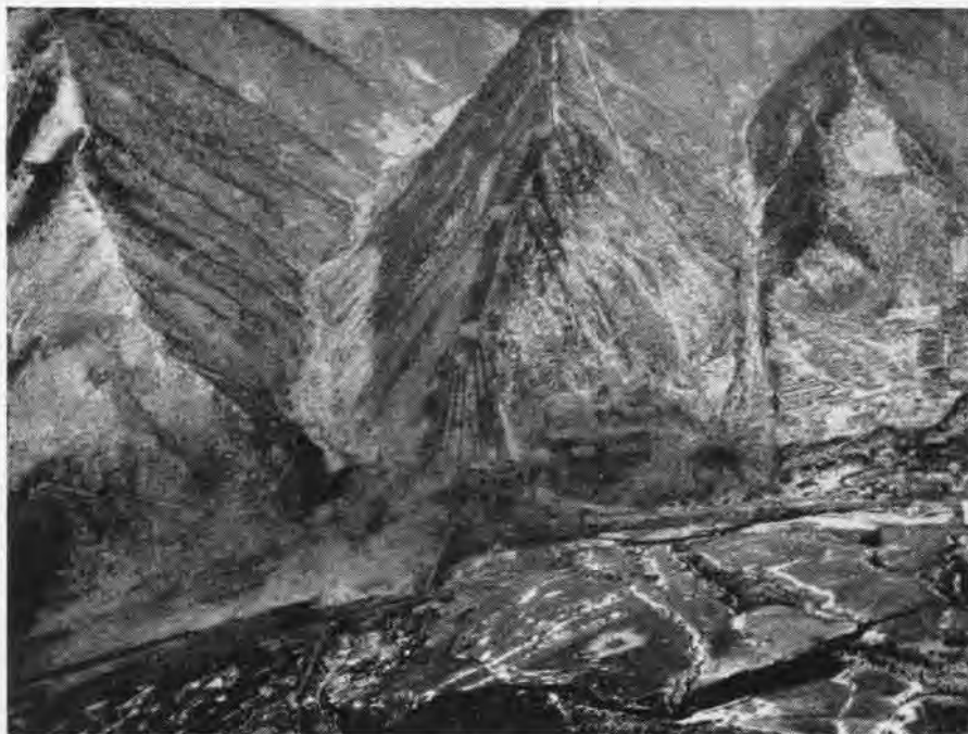
BLASTED generator building and demolished penstocks near Kyosen, North Korea left this area useless. Strike was made by CAG-7 pilots flying from Bon Homme Richard
