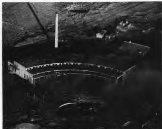
ESSEX bombs punched seven holes in reinforced concrete structure. It still stands as major force blasted down and inward
