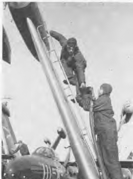
CARE REQUIRED IN HANDLING NEW JP JET FUEL
