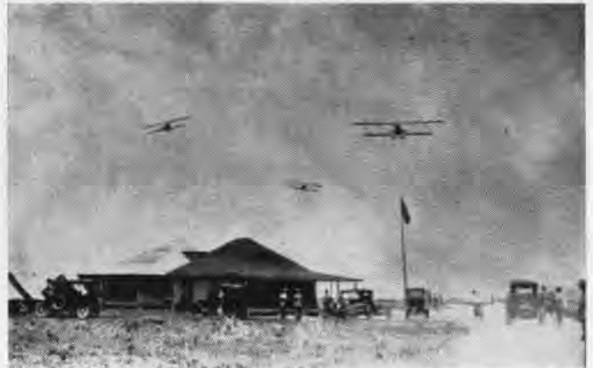
EARLY DAYS picture of MCAS Miami in 1918 shows Jennys flying over the administration building, still standing on the station
