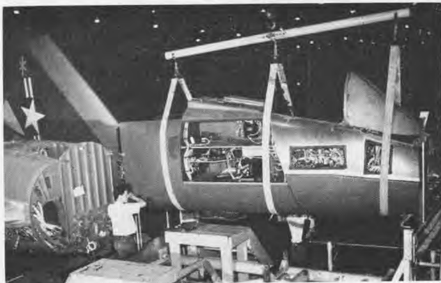
IAP PLANNING RESULTS IN NEW PRODUCTION AS REQUIRED. NOSE JOINS FUSELAGE
