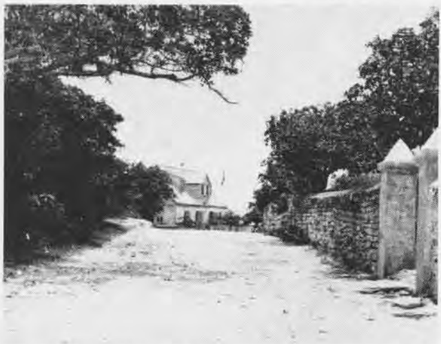
THE "PEACE and Plenty" Building at Georgetown with British flags flying stands at end of Bahamian road lined with trees and wall.
