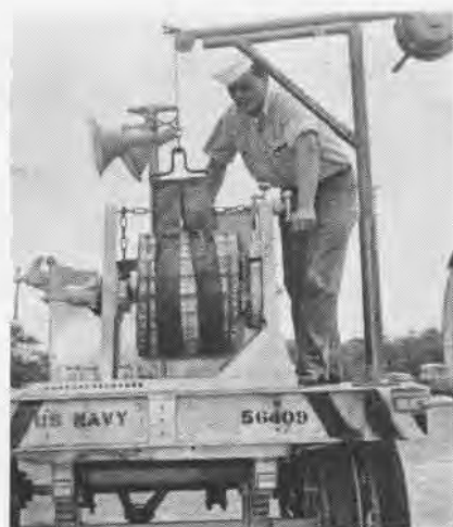
AT NAS Barber's Point , Charles E. Bloir, AO1, designed a labor-saving hoist which lifts tow cable reel on to re-wind truck. Here Bloir displays the results of his reel ingenuity.
