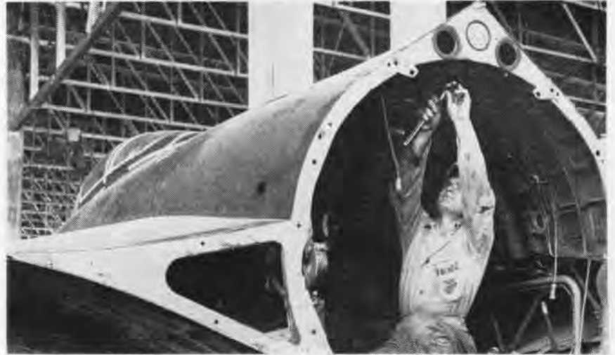
PFC GERAULD LANGUET STRIPS SCORCHED TAIL ASSEMBLY OF PANTHER FOR REBUILDING
