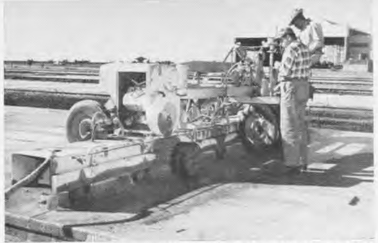
EXPANSION JOINTS MUST BE SEALED AGAINST MOISTURE JOINT SAWING MACHINE IN OPERATION AT MIRAMAR PLANE PARKING AREA
