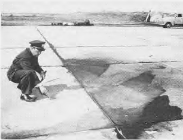
SCALED AREA AND MELTED JOINT FILLER RESULT OF JET BLAST JET BLAST HAS GOUGED SHOULDER OF SANFORD WARM-UP APRON
