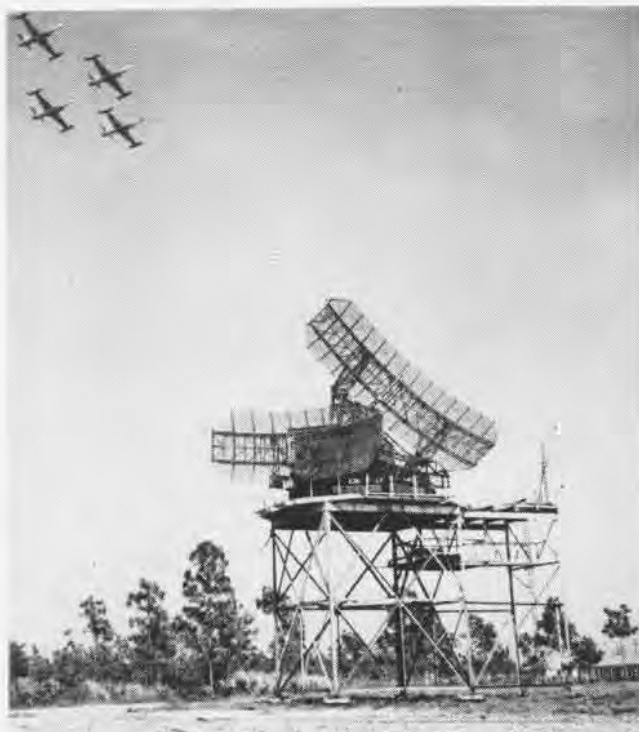
AS THE antennas of a huge, revolving CPS-6 radar system send out probing beams, F-94 interceptors speed on practice ADIZ mission.
