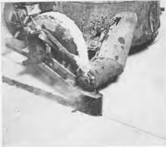
EXPANSION JOINTS MUST BE SEALED AGAINST MOISTURE JOINT SAWING MACHINE IN OPERATION AT MIRAMAR PLANE PARKING AREA
