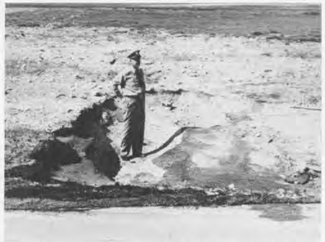
SCALED AREA AND MELTED JOINT FILLER RESULT OF JET BLAST JET BLAST HAS GOUGED SHOULDER OF SANFORD WARM-UP APRON
