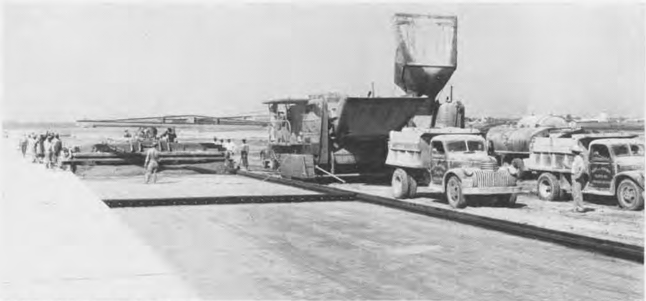
GOOD SUBGRADE WILL PREVENT CONCRETE SURFACE FROM SAGGING, BUCKLING, AND WILL SUSTAIN WEIGHT OF FAST-SINKING JETS
