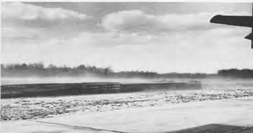
TWO-FOOT LONG ANCHOR BARS FAILED TO HOLD MARSTON MAT AGAINST BLAST OF JET
