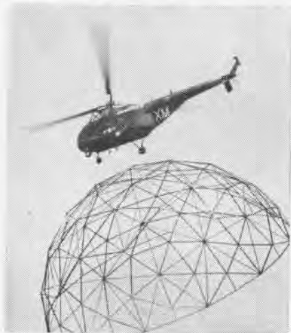
THE DOME CAN BE MOVED BY HELICOPTER
