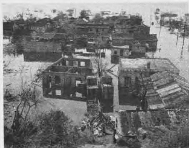
SCENES LIKE THIS one were typical of those sighted during the rescue work. Roofs were swept away and waters still stood in the streets.
