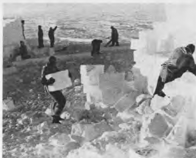
PLANES' HANGARS BUILT OF SNOW BLOCKS, ANTARCTICA, 1940
