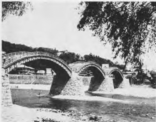
KINTAI Bridge, near Iwakuni, is one of the wonders of the Far East. Hornet sailors marveled at this example of Oriental Engineering.
