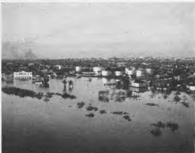
AFTER JANET passed south of Tampico, flood waters swirled in from the Tamese River to cover everything with a heavy coat of dirt.
