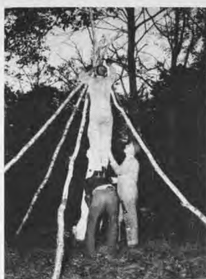
FIRST STEP IN ERECTING TEEPEE SHELTER
