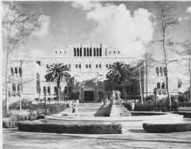
DOHENY LIBRARY FACILITIES ARE USED BY SAFETY STUDENTS
