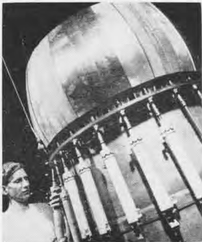
PNEUMATIC pistons are being installed that will regulate the aperture located in the rear.
