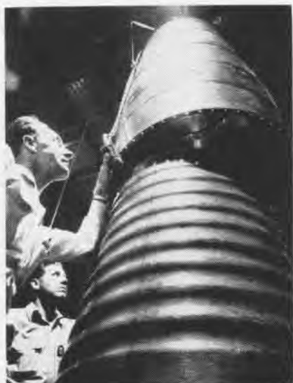
AN OUTER liner is lowered into place for use in combatting jet's extremely high temperatures.
