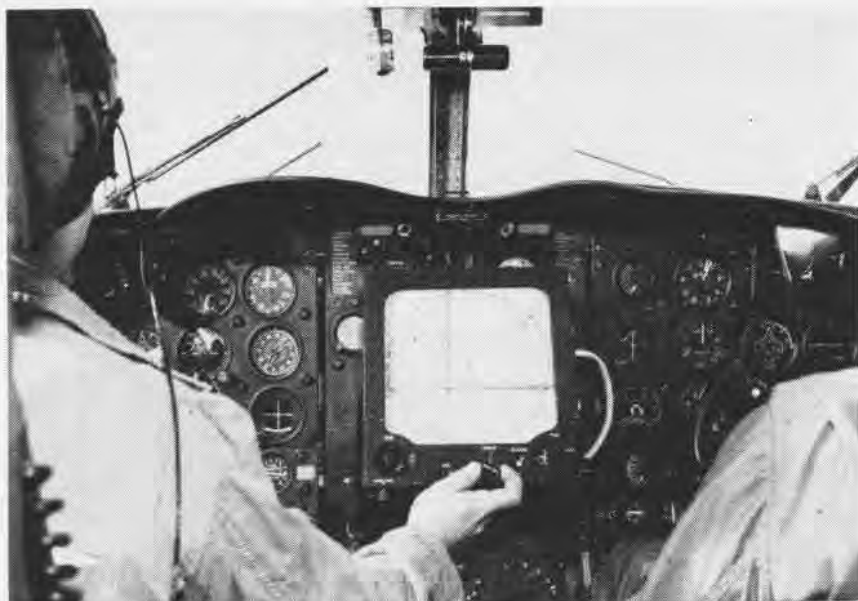
AUTOMATIC DEAD RECKONING NAVIGATOR "PADRE" GIVES THE PILOT A CONTINUOUS FIX
