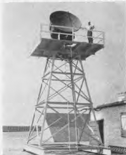
EYE OF Radar Weather Detection is perched on top of a special tower on roof of hangar.
