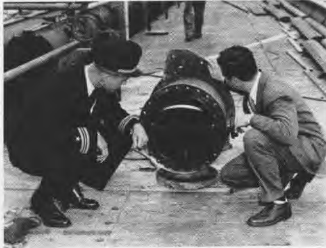
OFFICER INSPECTS EXHAUST TEE FLANGE WITH G. L. FERRIS
