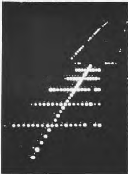
HIGH INTENSITY approach lighting systems have been installed in all major airports operated by Canada's Department of Transport, Civil Aviation Division. The one shown above, standard for RCAF fields, is known as the modified Calvert system. The Civil, or modified Alpha, system, is similar with a center line and crossbar light pattern and is standard for civil aviation.
