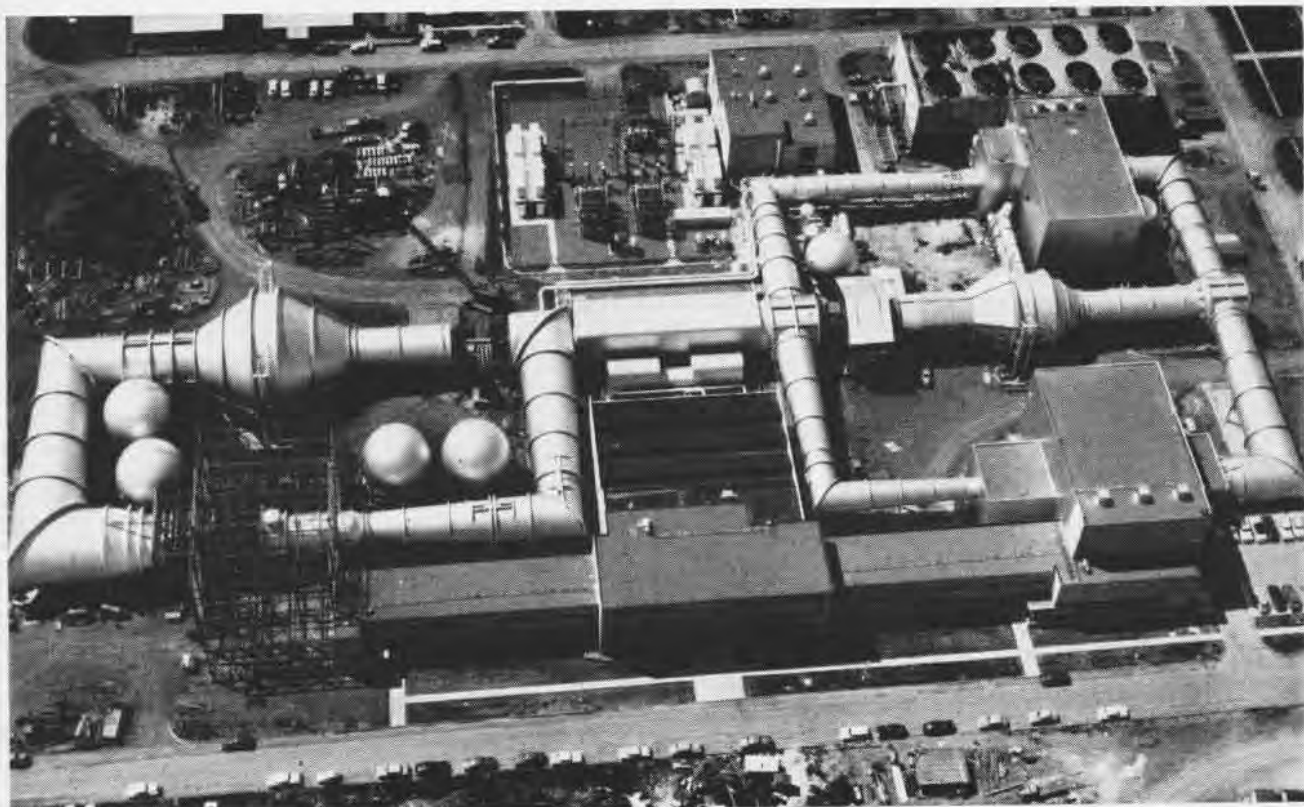
AMES UNITARY Plan Wind Tunnel covers 11 acres. It is a continuous flow tunnel in which three separate test sections cover speeds of
