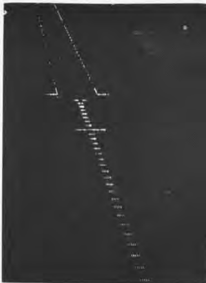
HIGH INTENSITY approach lighting systems have been installed in all major airports operated by Canada's Department of Transport, Civil Aviation Division. The one shown above, standard for RCAF fields, is known as the modified Calvert system. The Civil, or modified Alpha, system, is similar with a center line and crossbar light pattern and is standard for civil aviation.
