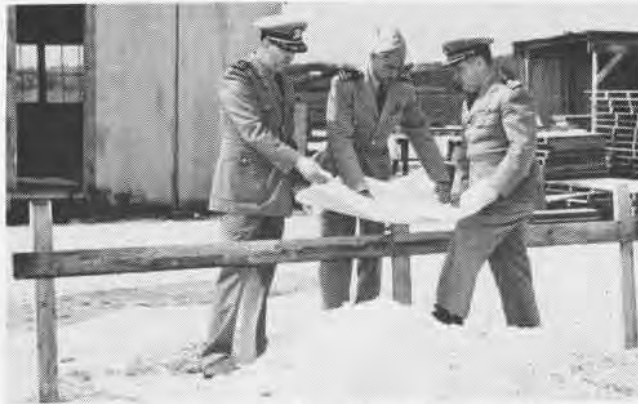
ACORN CEC Cdrs. Gray and Healey make on-the-spot study of construction plans with Lt. P. R. Jusper, Bermuda NavSta Public Works Officer.
