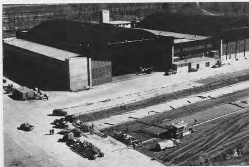
PARAMOUNT PROJECT OF THE GIGANTIC STATION RECONSTRUCTION IS MIRAMAR HANGAR
