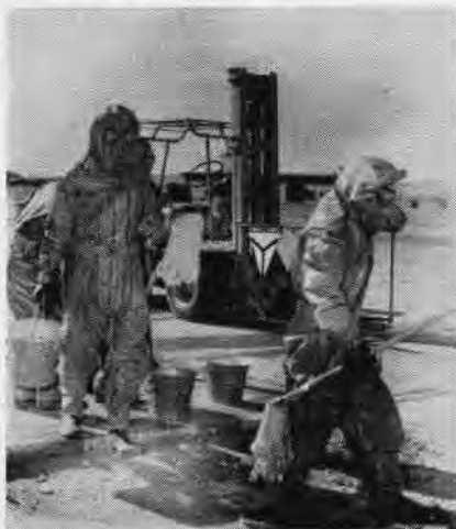
CREW IS READY WITH SWABS AND BUCKETS
