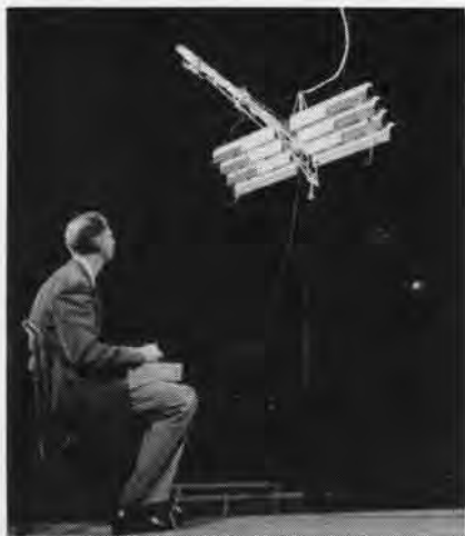
VERTICALLY rising model shown in hovering flight at the Langley Aeronautical Lab.
