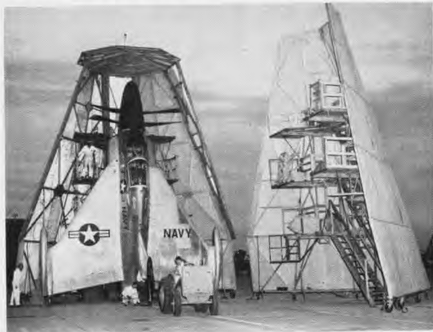
A MOTORIZED mule maneuvers the Navy's XFV-1 Pogo into position for housing in its unique hangar at NAAS Brown Field near San Diego. The tepee-shaped hangar on wheels enfolds the plane like halves of a clamshell and incorporates a triple-deck work platform for easy access to every part of the revolutionary new vertical take-off fighter. The Pogo's hangar is the smallest ever devised for a Navy plane. Built of steel framework and wood, the hangar is fire resistant.
