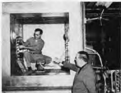
GEORGE LINK , electrician, is making final wiring changes on inverter to be tested.
