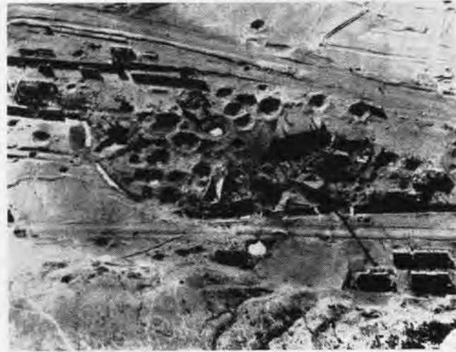
POST STRIKE damage assessment determined that area was destroyed. About 14 locomotives were in yard and shops when strike was made.
