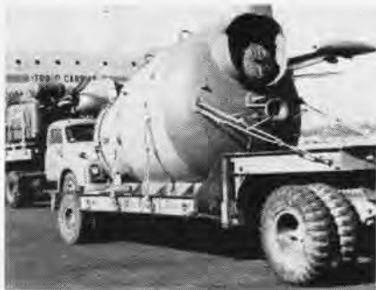
SUB GEAR AWAITS LOADING ON AF C-124
