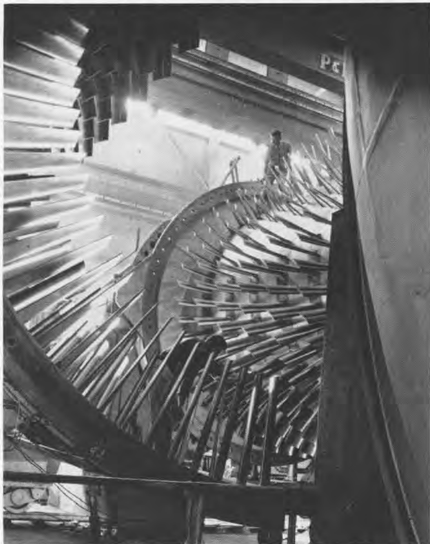
MAIN COMPRESSOR BLADES PROPEL 2000 POUNDS OF AIR PER SECOND THROUGH TUNNEL
