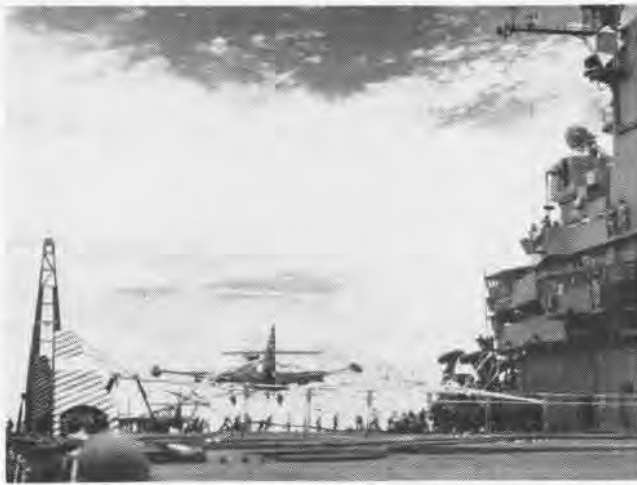
ARRESTING GEAR WAS BUILT BY NAVAL AIR ENGINEERING FACILITY
