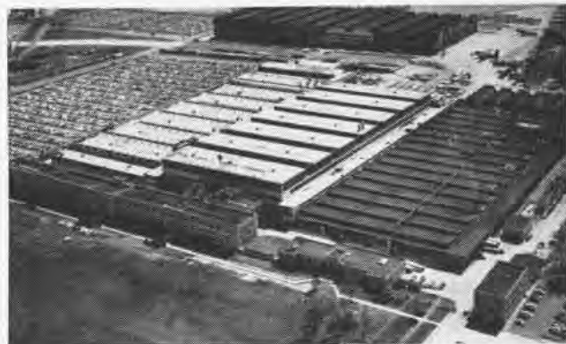
AERIAL VIEW OF THE MARTIN PLANT #1 AT MIDDLE RIVER, MD.
