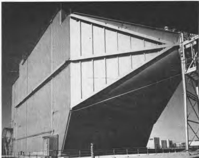
THIS IS THE AIR DRYER BUILDING OF LEWIS UNITARY PLAN WIND TUNNEL COOLED TUNNEL AIR IS DIFFUSED AROUND THIS CONE
