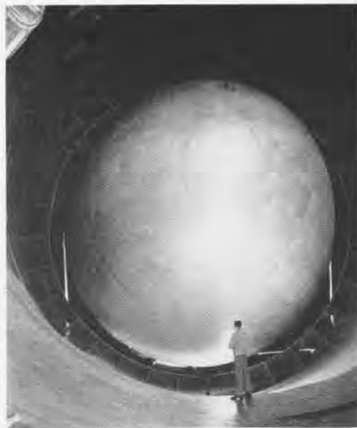
THIS IS THE AIR DRYER BUILDING OF LEWIS UNITARY PLAN WIND TUNNEL COOLED TUNNEL AIR IS DIFFUSED AROUND THIS CONE
