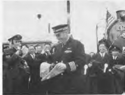
DONNING CAP and gloves of a Japanese Railroad engineer, Capt. W. E. Premo, CO of NAS Iwakuni, prepares to pilot the first train over new 2.5 mile spur that joins NAS to main line.
