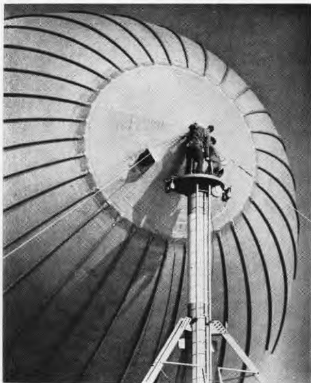
They are every day utilities for Navy. The 'N' type blimp, left, holds about 900,000 cu. ft. of helium when inflated.
