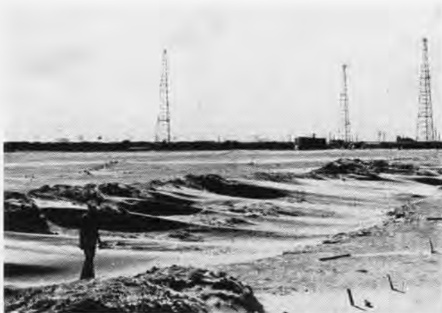
A GREAT AIR STATION WAS TO RISE ABOVE THESE SAND DUNES
