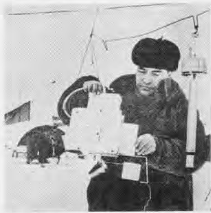
AEROLOGIST is important member of expedition. Here he checks radiosonde before release.
