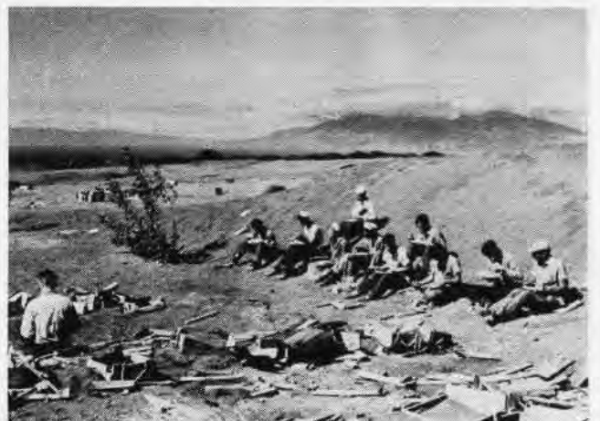
REFURBISHING the target range took the crew four days. Lt. O'Connell praised the men: "This is the hardest working crew I have ever seen."
