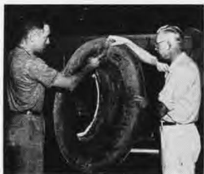
ALAMEDA workmanship is rated high. O&R employees inspect newly constructed venturi.
