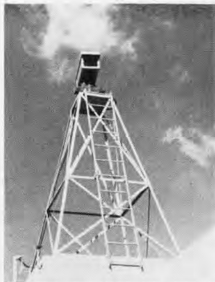
TV CAMERA INSTALLATION ATOP BLDG. 27
