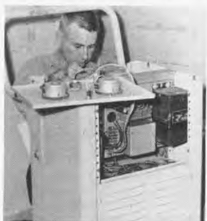
FIX-IT MAN C. C. Ulsh, AE1, repairs the rectifier unit to boost current required.
