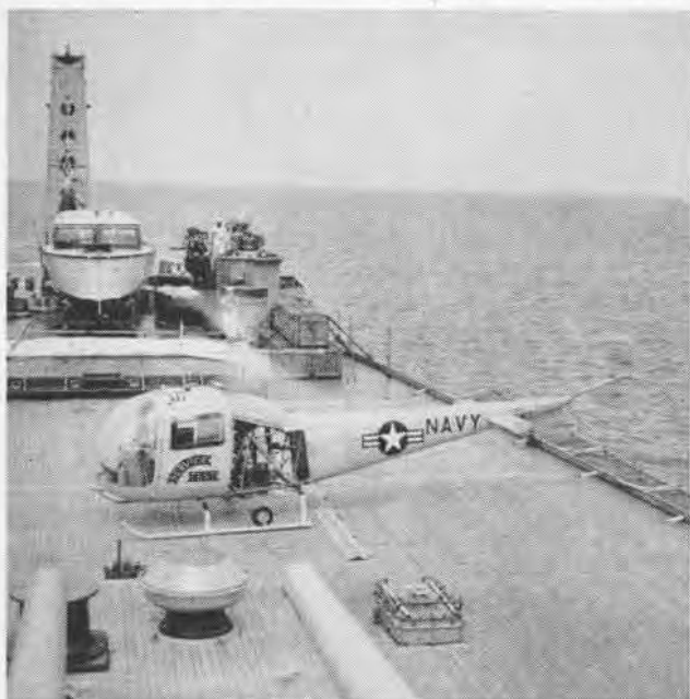
HUL-1 ON DECK OF NEWPORT NEWS DURING TESTS
