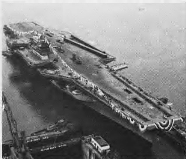
FORRESTAL IS REMOVED FROM DRYDOCK #10, NEWPORT NEWS, VA.
