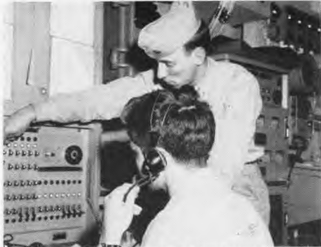
ENS. ZERBEL INSTRUCTS O'CONNOR ON SWITCHBOARD OPERATION
