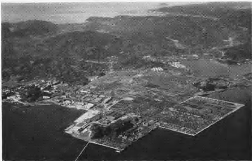
TWO WORLD wars and 45 years later, Oppama is now the site of the U. S. Naval Air Facility and the Army's Ordnance Command, Japan. Emphasis is now on support of the fleet repair program.
