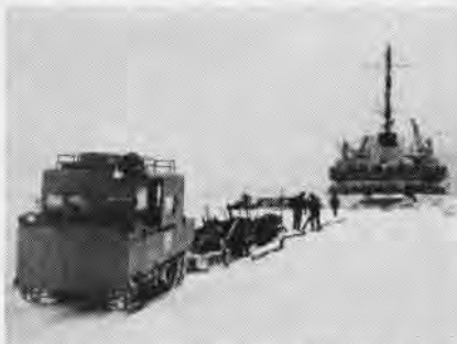
LAYING FUEL HOSE FROM AOG TO TANKS
