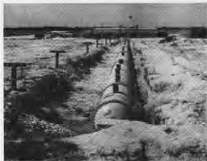
WATER TUBE INSTALLATION IN DELAWARE
