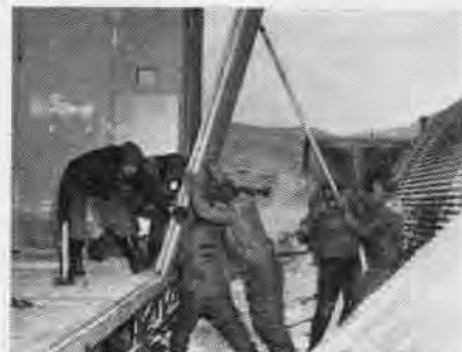
LIFTING PANEL IN PLACE WAS HEAVY WORK
