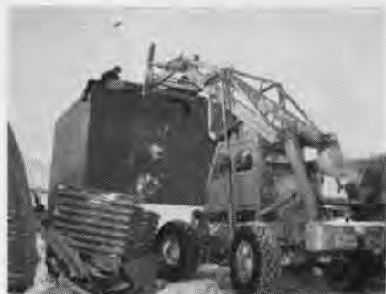
THE PETTIBONE LIFTS HEAVY ROOF PANEL
