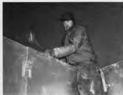
CLIPS, NOT NAILS, HELD PANELS FAST
