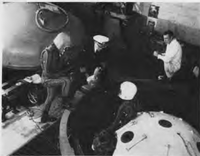
CLOSED GONDOLA and balloonists go for trial run in General Mills' "bean pot," a low pressure chamber simulating high altitude conditions.
