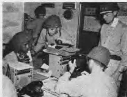
A 'NERVE CENTER' FOR THE REPAIR TEAMS
