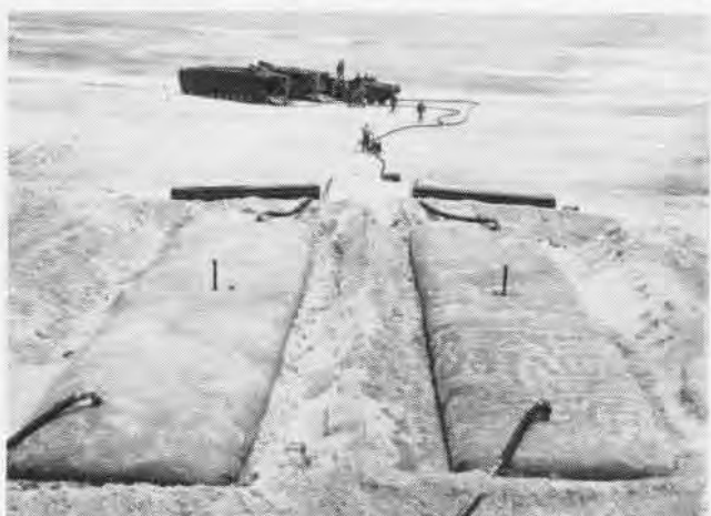
BEACH STATION keeps up fuel flow from land craft, through tanks, to field units. Tanks measure 12 feet long, 2.5 feet in diameter.
