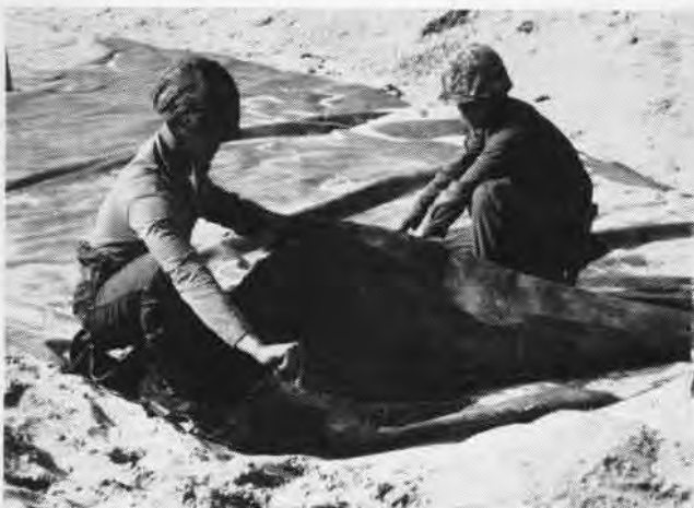
COLLAPSIBLE FUEL tank is unfolded as Marines set up a beach unloading station. Bag is easily unrolled and can be filled in minutes.
