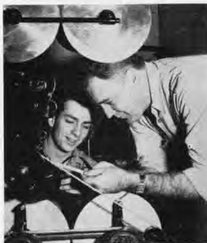
PHOTOGRAPHERS check Model-J movie printer which produces positive film from negative.
