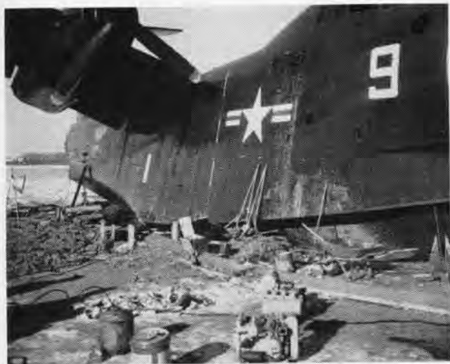
EQUIPMENT IS READY FOR THE CONSTRUCTION OF THE COFFERDAM
