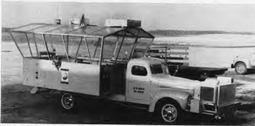
OVER-ALL VIEW OF ATU-206'S TRUCK-MOUNTED, MOBILE CONTROL TOWER, THE 'THANG'
