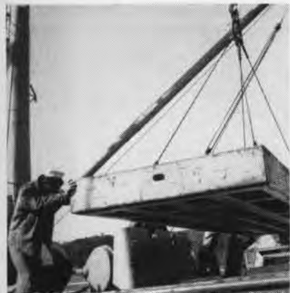
AFTER UNLOADING, MEN CLOSE HATCHES
