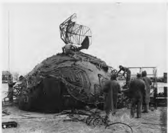
HUT TAKES SHAPE QUICKLY AFTER DELIVERY TO TRAINING SITE
