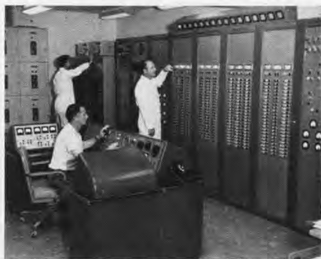
CENTRAL CONTROL ROOM OF NOTS AEROBALLISTICS LABORATORY
