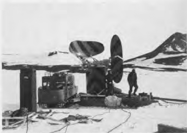
GCA UNIT PUT ON GO-DEVIL SLED FOR TOWING TO SEA-ICE STRIP
