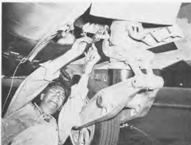
NEW NOSE GEAR CENTERING DEVICE IS INSTALLED AFTER TEST
