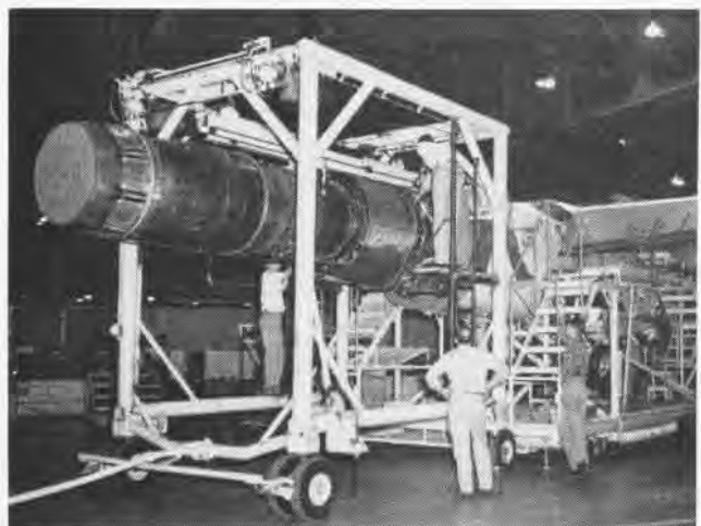
NEARING END OF ASSEMBLY LINE, POWER PLANT IS INSTALLED
