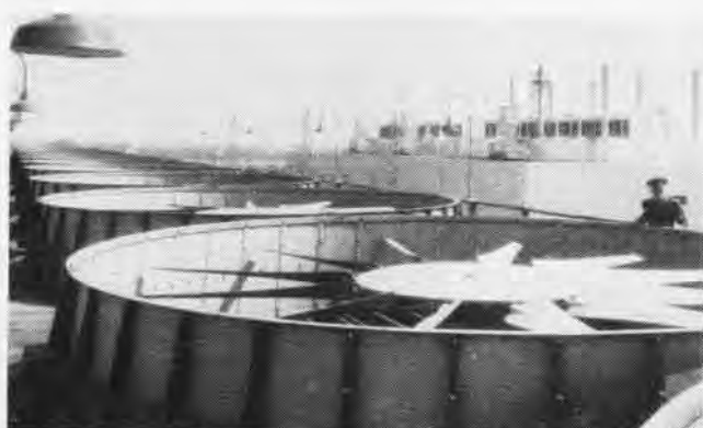
GIANT FANS WASH HEAT FROM WATER AND PERMIT ITS RE-USE
