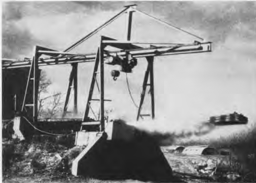
6000-POUND DEADLOAD IS FIRED FROM A SCALE SIZE MODEL OF THE C-14 CATAPULT
