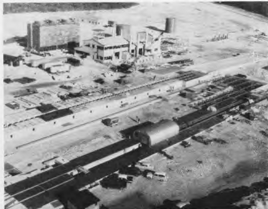
C-14 CATAPULT (FOREGROUND) BEING INSTALLED AT LAKEHURST. NOTE C-13, CENTER
