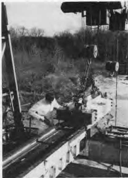
DEADLOAD SIMULATES WEIGHT OF AIRCRAFT
