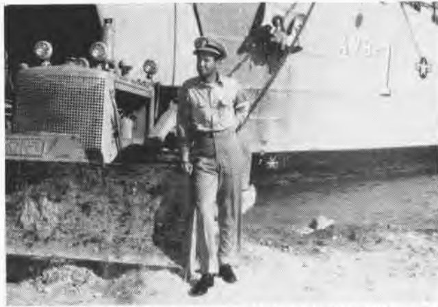
PRESENT C.O. , Cdr. Sinclair leans on blade of bulldozer, first piece of equipment to leave ship when remote airstrip requires activation.
