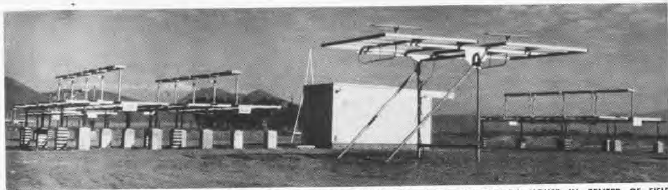
PART OF THE ANTENNA FIELD AT NAAS BROWN FIELD SATELLITE TRACKING SITE. NOTE THE CAMERA HOUSE IN CENTER OF FIELD
