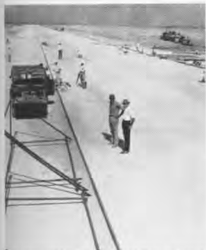
FOUR-THOUSAND FT. TAXIWAY BEING BUILT
