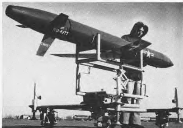
TEAL LENGTH, 12 FT.; DIAMETER, 10 IN.; WING SPAN, 58.8 IN.
