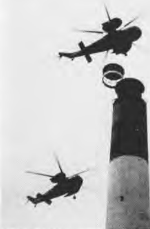
SECOND MARINE Air Wing helicopters lift a 1740-pound lantern to the top of Oak Island Lighthouse near the mouth of Cape Fear River at South Port, N. C. The operation helped complete first area lighthouse in 54 years.
