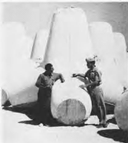
25-TON 'TETRAPODS' FOR THE BREAKWATER
