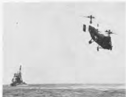
HSL-1 TOWS 300-TON FLOATING DERRICK
