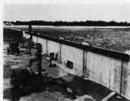
13,000,000-GALLON RESERVOIR TRAPS RAIN
