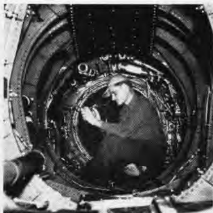
ELECTRICIAN CHECKS WIRING OF A FURY
