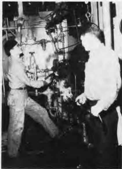
CAT BOILER is lighted. It takes 1½ hours to produce 600 lbs. steam per square inch.
