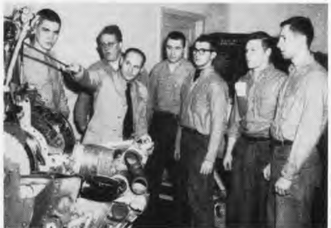
CUTAWAY OF an AD engine is explained by Chief Miller at NAS Moffett Field to members of Grosse Ile's Fascon 731 training there.
