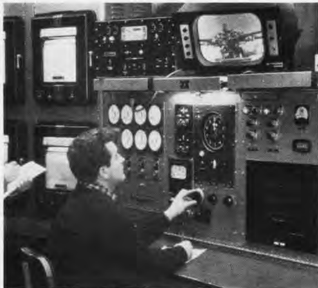
THE WORLD'S LARGEST helicopter whirl test stand known to be in existence is now in full operation as Sikorsky Aircraft Division of United Aircraft Corporation, Stratford, Connecticut. The king size facility (R) has been in the process of design and construction five years. To the left of the cone-shaped, steel plated stand are elevators used to carry personnel and huge rotor blades to the top of the stand.
