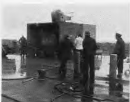
FIRST RUN of new Kittell Lacy jet engine-test cell at NAS Whidbey Island is watched by crash crew and station fire department. Cell, which can handle engines up to 30,000 pounds thrust, will be used by FASRON 112.
