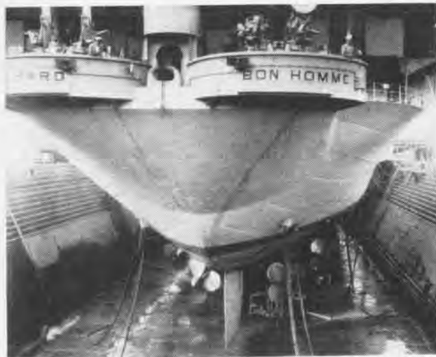
FANTAIL BEFORE TWO 3" 50 MOUNTS AND TUBE WERE REMOVED
