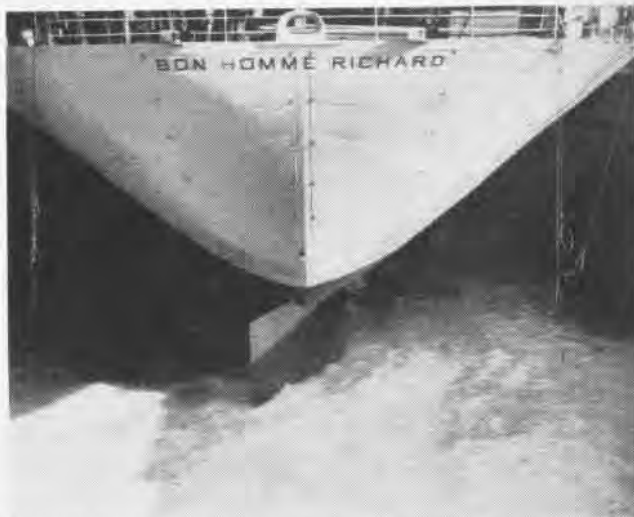
FANTAIL AFTER REMOVAL AS WATER FLOWS INTO THE DRY DOCK
