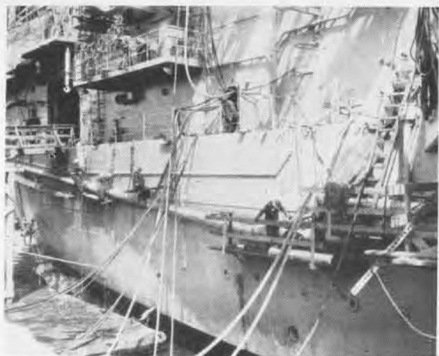
BARGE LINES, WORK BOOMS, LADDERS, SIGNIFY MEN AT WORK
