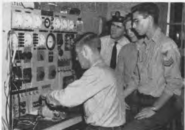
CENTER HANGAR ELECTRICIANS CHECK INVERTER WITH VARIDRIVE
