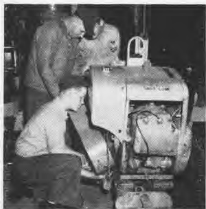
OVERHAUL STARTED ON AIR COMPRESSOR
