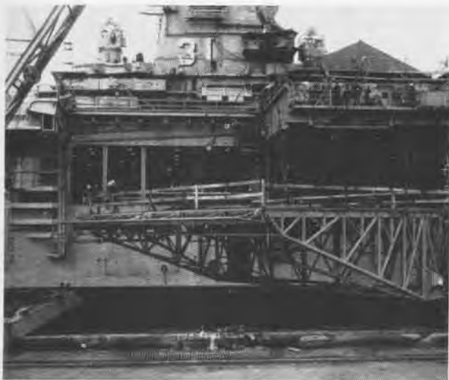
YARD CRANE SWINGS LENGTHENED NO. 2 ELEVATOR INTO PLACE
