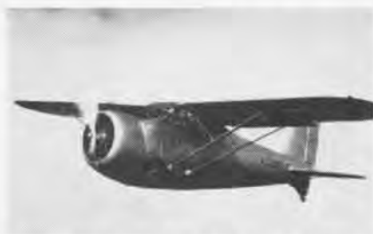
IN XF13C, CABIN REPLACED OPEN COCKPIT
