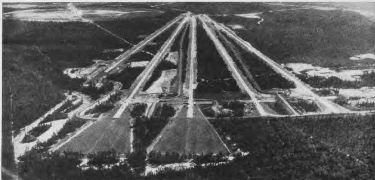
AIR VIEW SHOWS PREVIOUSLY COMPLETED TRACK, LEFT, AND FOUR NEW TRACKS. NAS IS IN BACKGROUND, OUT OF VIEW AT TOP
