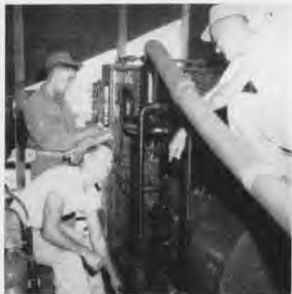
SSGT. CHARLES FLEMMING (R), directs operation of liquid oxygen plant on Marine airstrip in southern Formosa. LOX plant was airlifted to Formosa where it is used for jet aircraft high altitude breathing apparatus.
